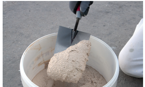
2. Remove the PX-28 Isolxtrem SILOXANE TECHNOLOGY M with the help of a pallet.
