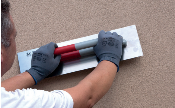
5. Smooth the PX-28 Isolxtrem SILOXANE TECHNOLOGY M
