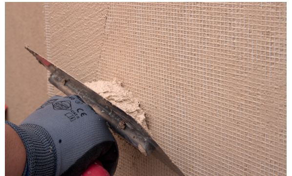
8. Cover the screen with PX-28 Isolxtrem SILOXANE TECHNOLOGY M
