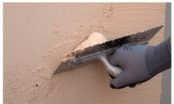
4. Apply PX-28 Isolxtrem SILOXANE TECHNOLOGY M on the surface.
