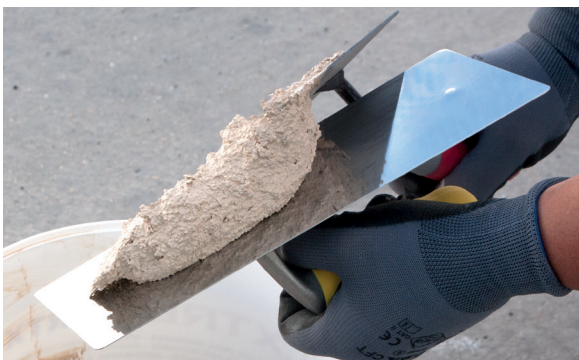
3. Place PX-28 Isolxtrem SILOXANE TECHNOLOGY M on the trowel.
