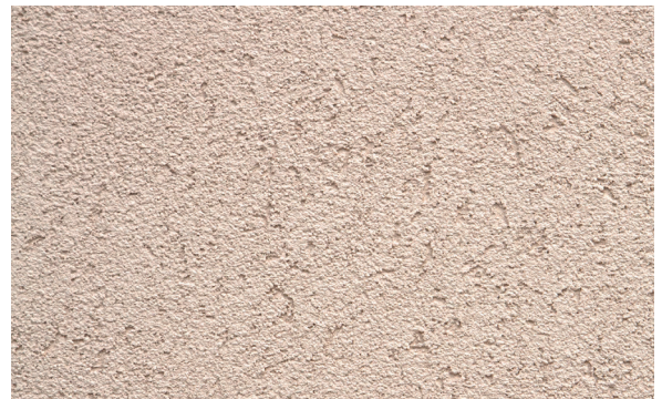
10. Final finishing of the PX-28 Isolxtrem SILOXANE TECHNOLOGY M
