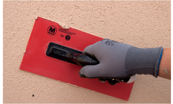
6. Trowel the PX-28 Isolxtrem SILOXANE TECHNOLOGY M
