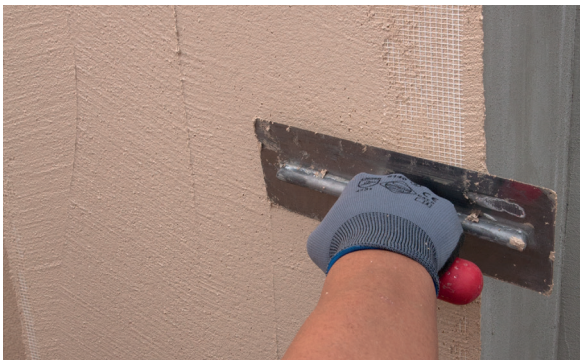
9. Smooth the PX-28 Isolxtrem SILOXANE TECHNOLOGY M deposited on the mesh.
