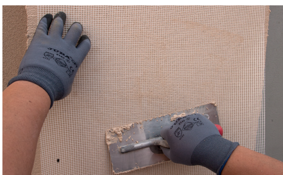
7. Colocar la malla RG-116 Isolxtrem System.
