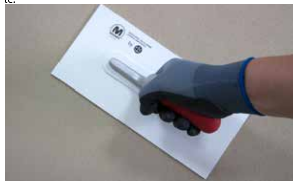
6. Espatular o PX-28 Isolxtrem SILOXANE TECHNOLOGY F.
