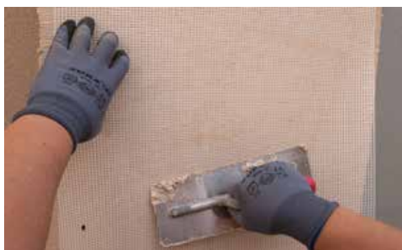
7. Colocar a malha RG-116 Isolxtrem System.
