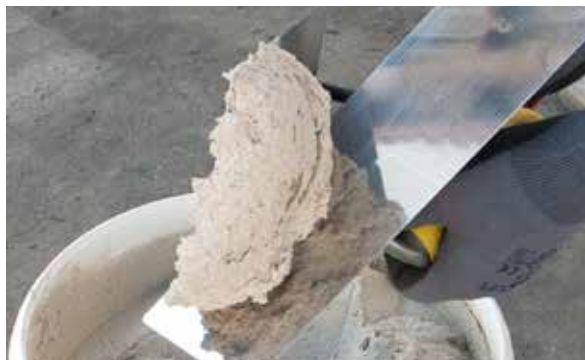
3. Coloque PX-28 Isolxtrem SILOXANE TECHNOLOGY F na espátula.
