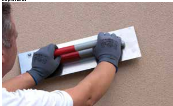
5. Alisar o PX-28 Isolxtrem SILOXANE TECHNOLOGY F.
