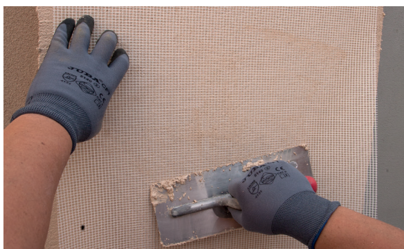
7. Colocar la malla RG-116 Isolxtrem System.
