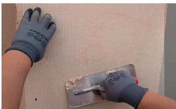
7. Colocar la malla RG-116 Isolxtrem System.
