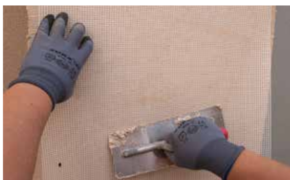
7. Colocar a malha RG-116 Isolxtrem System.
