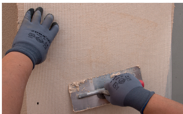
7. Colocar la malla RG-116 Isolxtrem System.
