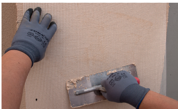
7. Colocar la malla RG-116 Isolxtrem System.
