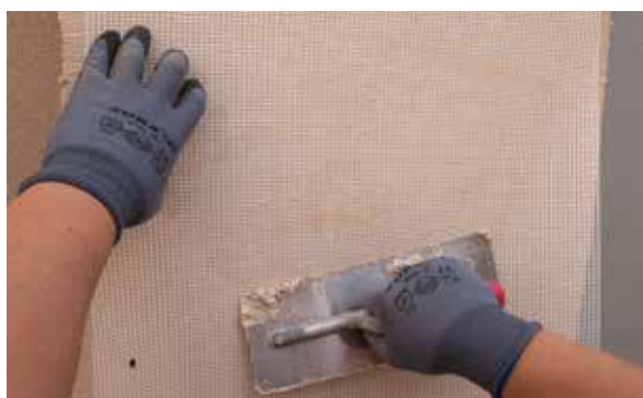
7. Colocar a malha RG-116 Isolxtrem System.
