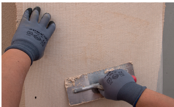
7. Colocar la malla RG-116 Isolxtrem System.
