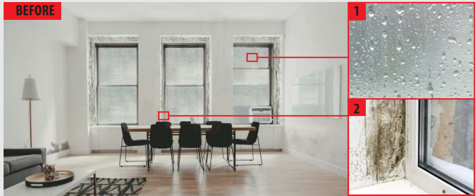
1. Drops of water produced by condensation. 2. Mold stains.
