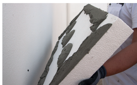
6. Placing the panel on the surface
