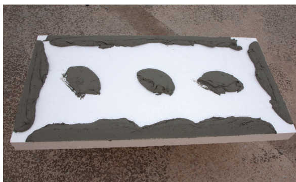
5. EPS panel gluing
