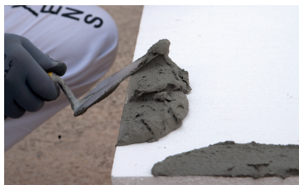
4. Application of CX-41 Colbaixtherm on EPS
