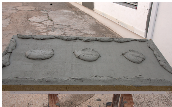
8. Placement of the rock wool board
