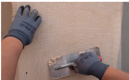
7. Colocar la malla RG-116 SolxTrem System
